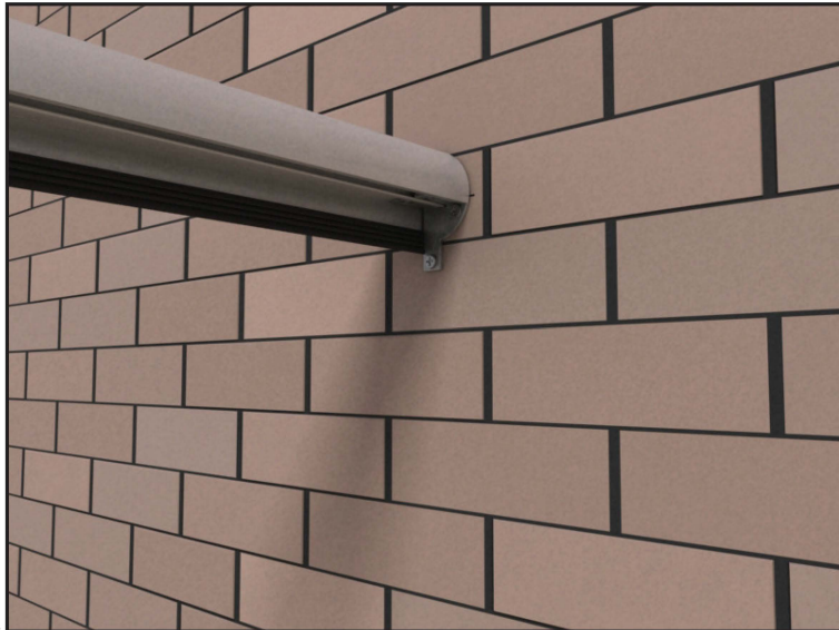
21 Drop the handrail onto the angle bracket
