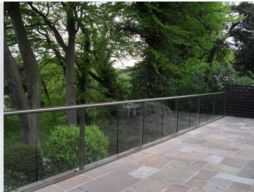
Balcony 2 Balustrade on a public roof terrace
