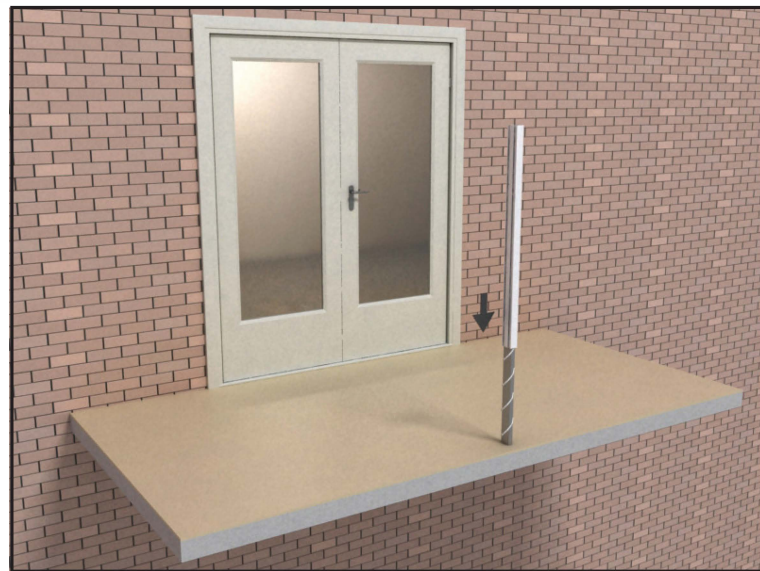
16 Slide the system cover post onto the primary post
