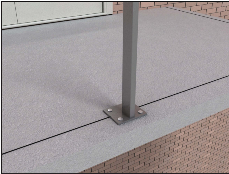
13 Use the appropriate fixings (Post fixing can be done at primary stage by locating the posts using measurements)
