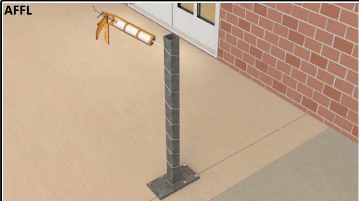
18a) Apply a thick bead of high quality neutral silicone around the primary steel post in a spiral fashion.
